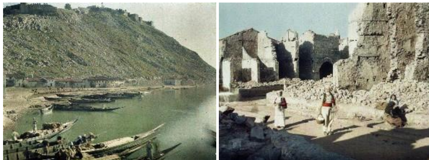
Figure 10.1 Castle of Shkodra and the customs in Bune / Figure 10.2 The walls of the castle from inside, showing the destruction after the war also of the Saint Stephen's Church wall
